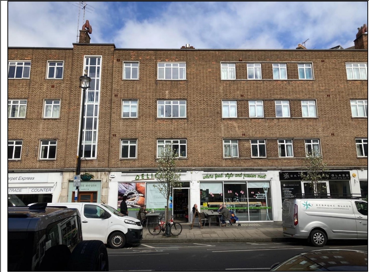
Front view of application site
